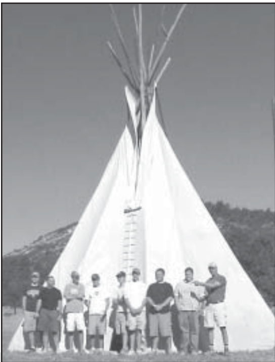
An important element for a Pow Wow is an authentic teepee. Some of the volunteers from Pelham Road erected this one under the leadership of one of the Native American elders. The poles were 30 feet long and heavy. They were woven together at the top with a heavy-duty rope. Then a tremendous canvas "skin" was used to wrap the structure and create the shelter.
